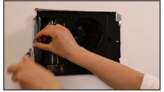
5. Remove the screw on the heater assembly and carefully remove it from the wall can.
