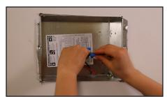
7. Line up the wires from the new heater and twist the wire connectors until tight. Pull each wire to ensure a good connection.
