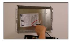
6. Disconnect the wires from the original heater.
