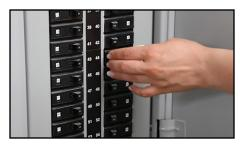
1. From the breaker panel, turn off the power to the heater.
